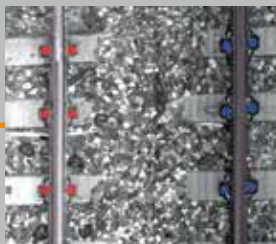
Elastic Fastener Inspection
