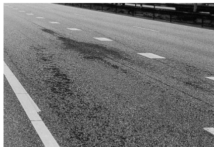
Figure 14. Example result of sealed cracks detection
