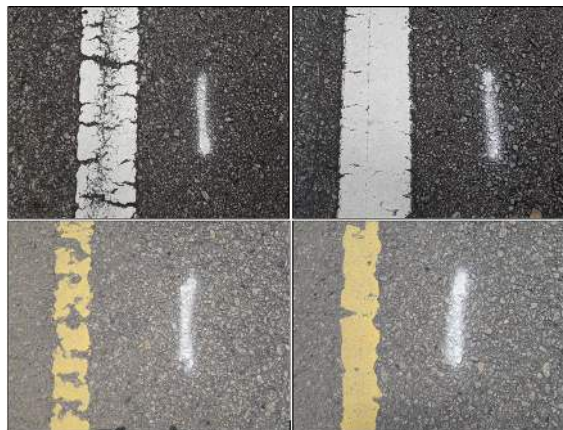
Fig. 5 Selection of different levels of wear
