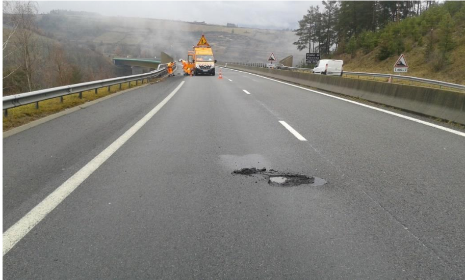
Figure 1 : Potholes occurring on the road.
