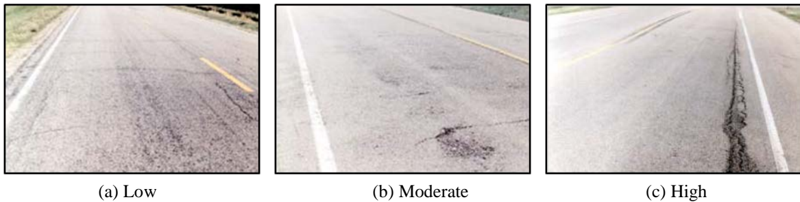
FIGURE 3 Raveling classification in NDOR (NDOR 2002).
