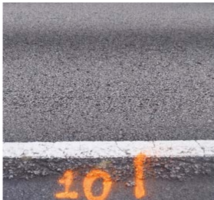
FIGURE 34 Typical pavement surface on test section #4.
