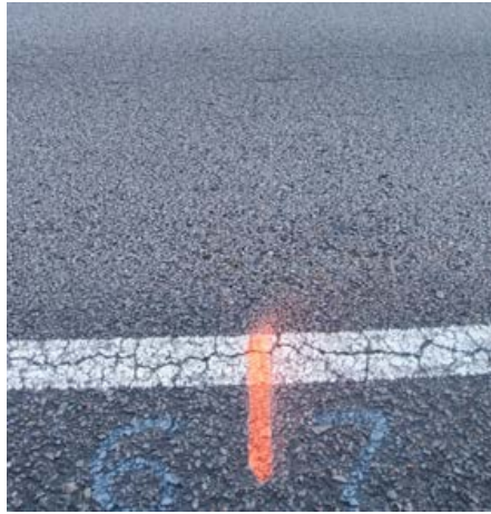
FIGURE 33 Typical pavement surface on test section #3.
