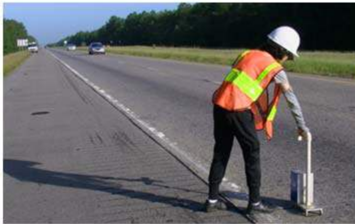
(b) Manually measure faulting on the roadway
