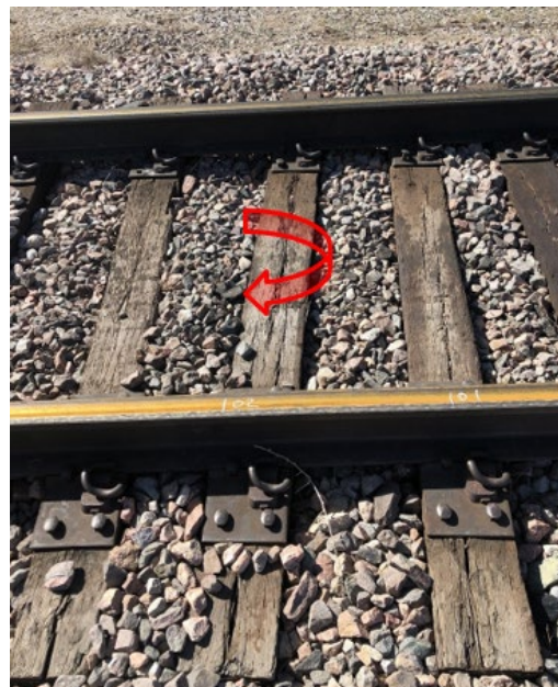
Figure 31. Timber Crosstie Skew Example
