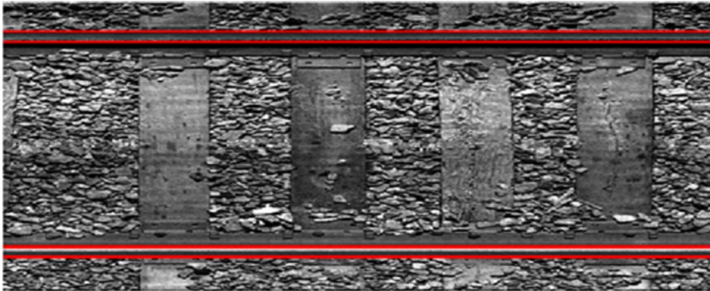
Figure 18 Detection and localization of the rail positions.
