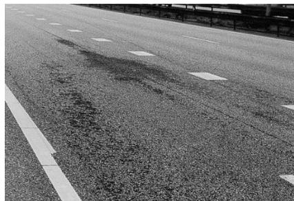
Figure 14. Example result of sealed cracks detection
